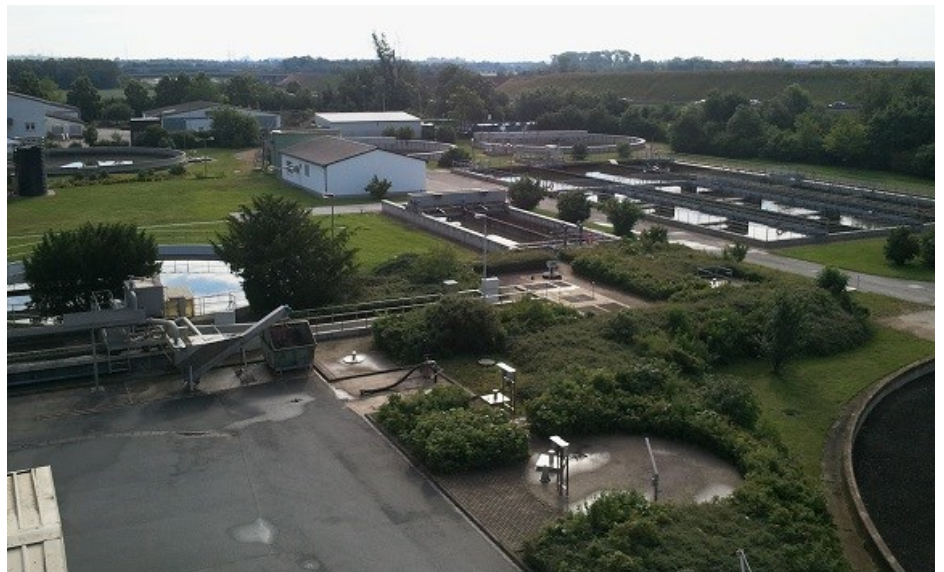
Wastewater treatment plant Ginsheim-Gustavsburg
